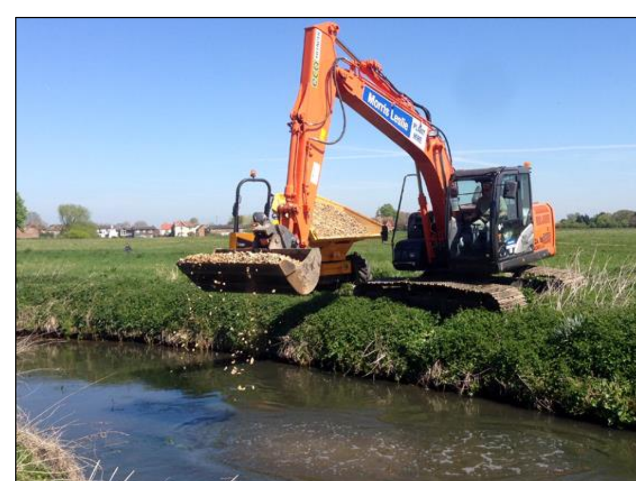
Initial construction occurred using heavy equipment
